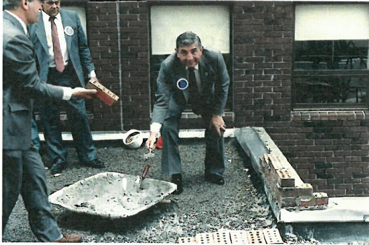
Parish Council President Tracy Demos at bricklaying for three new classrooms.
