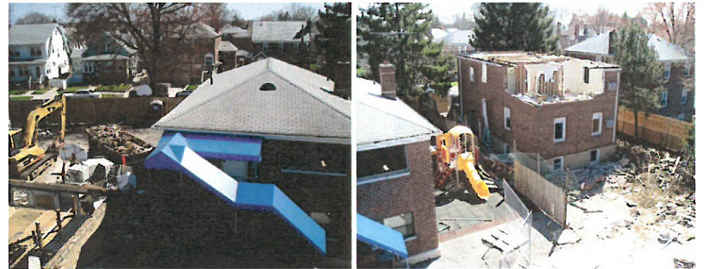
Preparing for Construction
