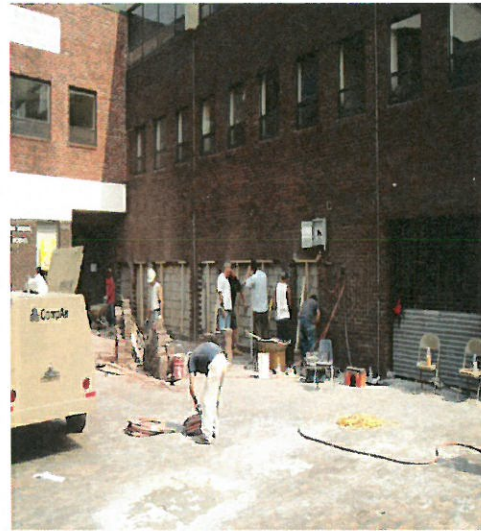
Preparing to create the Doulaveris Nursery School
